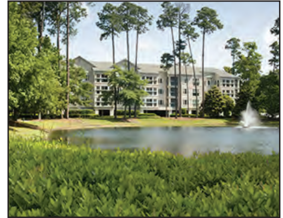
Main Building Exterior
